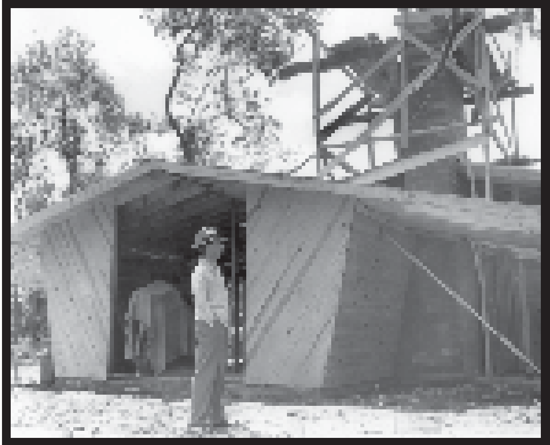
Alden B. Dow, Herbert Henry Dow, founder of Dow Chemical Company, moved to Freeport at the request of Dr. Beutel to design and supervise the construction of Lake Jackson. Alden stands watch over the construction of his office, and the first permanent commercial building constructed in Lake Jackson. The building now serves as the Alden B. Dow Office Museum after it was saved from demolition and restored to its original 1943 design in 2007 by the Lake Jackson Historical Association.
